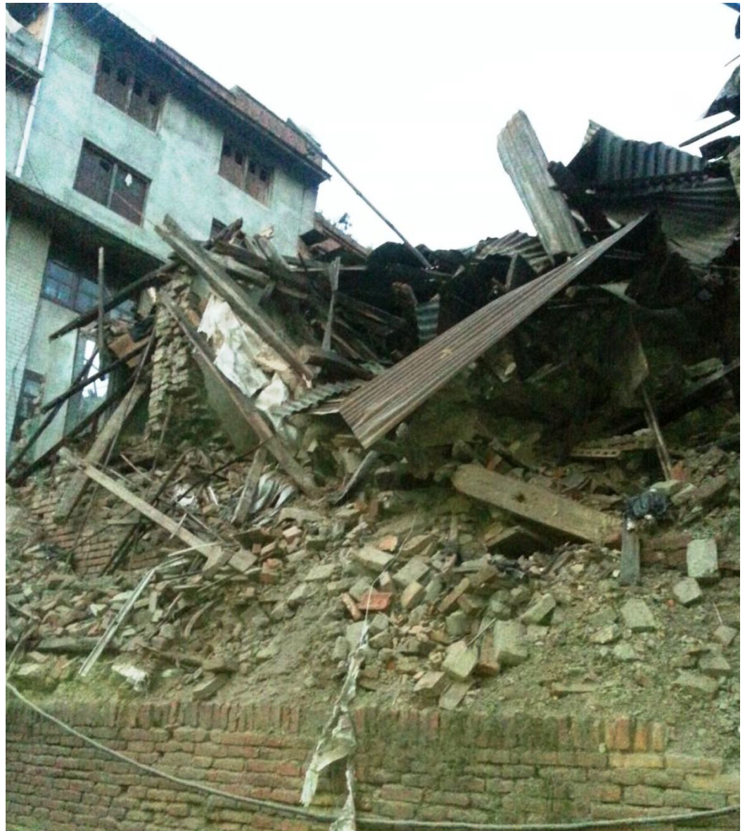
FIGURE 2: Severely damaged and collapsed buildings mainly responsible for injuries.
